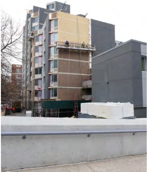
Top: Center pathway within complex to school. Bottom: EIFS being applied over the original ribbed-concrete block. Nov. 2021
